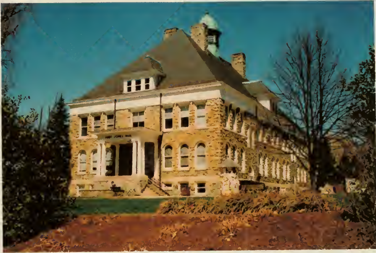
Photograph #40: The Model School (1899), also known as the Demonstration School, West Chester Normal School, now West Chester University, in West Chester Borough. The serpentine for this building came from Brinton's Quarry in Westtown Township.
